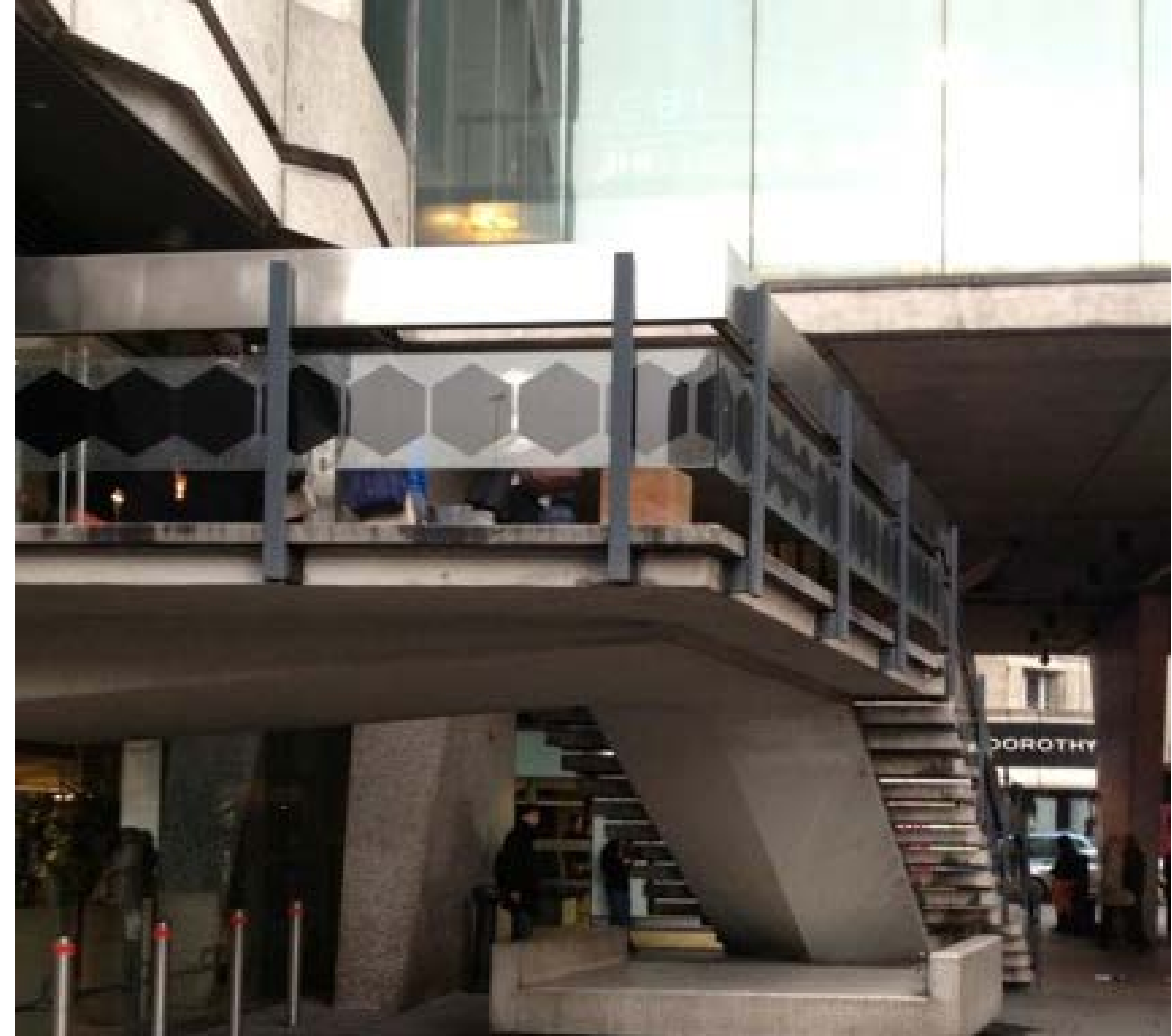
BEFORE EXTERNAL ACCESS STAIRCASE
